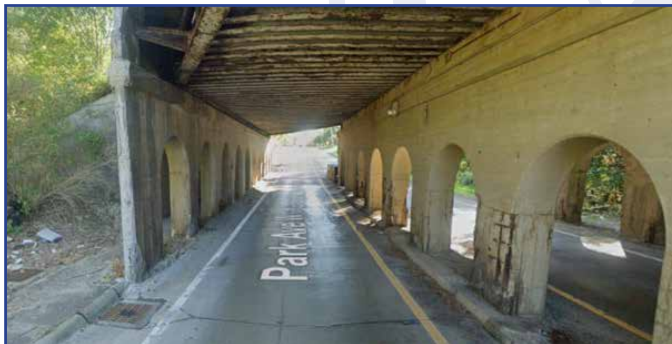
Streetview of an underpass at Park Ave.
