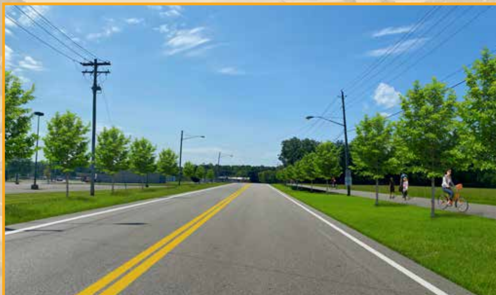
Connecting residents to key community assets is important in the Lexington-Springmill area but current connectivity options for pedestrians and cyclists are limited. This rendering depicts Stumbo Road behind the entrance to the Richland Mall repurposed as a two-lane road with a shared use path running along the western side of the right-of-way.
