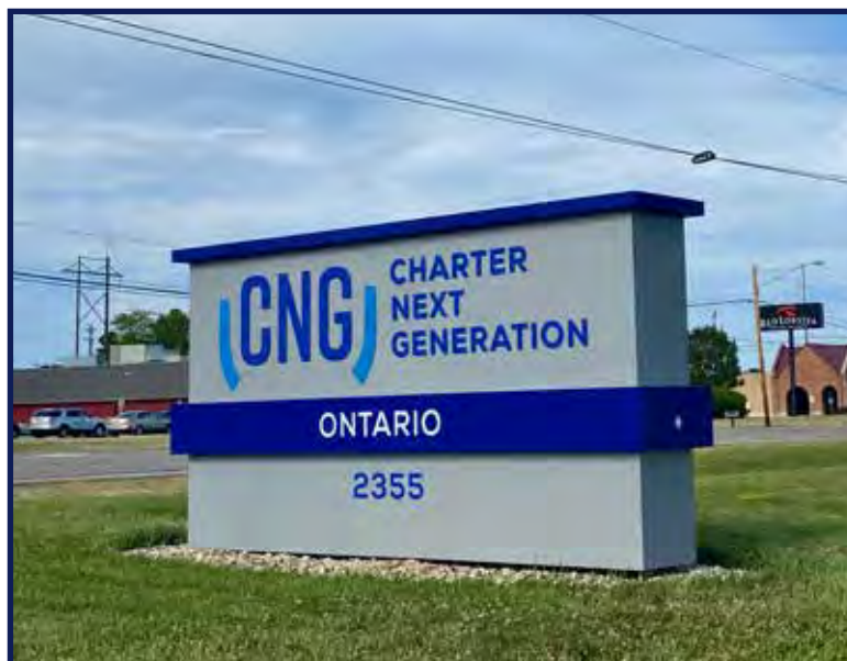
Charter Next Generation began operations on a part of the former General Motors site in 2021.
