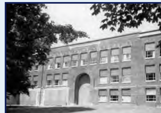
The former Springfield Township School/Ontario Junior High School.
