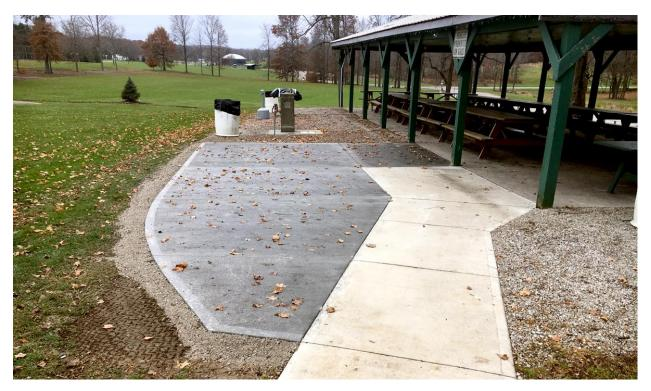
We received a complaint on the sidewalk at the corner of Park Avenue West and Briggs Drive. Part of the sidewalk on the Northwest corner sunk down, causing it be uneven. That part of the sidewalk was removed and leveled.
